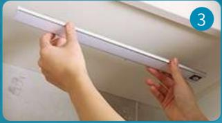
Make sure the installation surface is clean and smooth and place the light with mounting brackets onto the surface.
